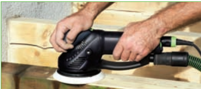
For coarse sanding of weathered beams.
